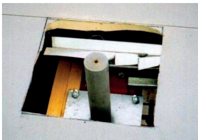
Traditional 'through the roof' post
